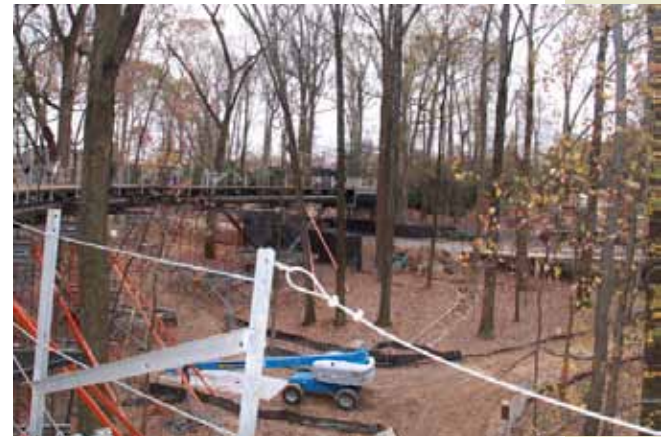
Arboguard's tree preservation work in progress
